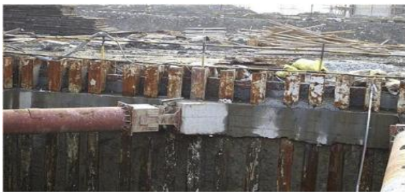
Figure 1. Constructed DSMW used in a subway project in Tianjin, China
